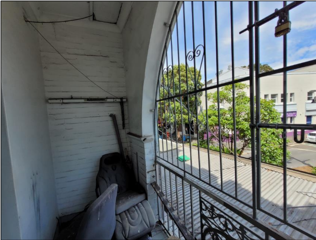
Figure 13: View of the front balcony of No.610
