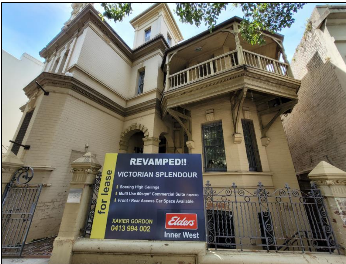
Figure 4: View of the heritage item at No.594-596, from Crown Street
