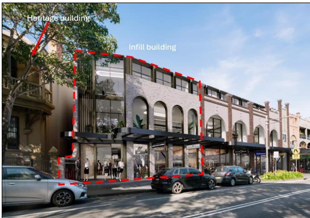
Figure 55: Crown St perspective of the original scheme submitted as part of the current application
